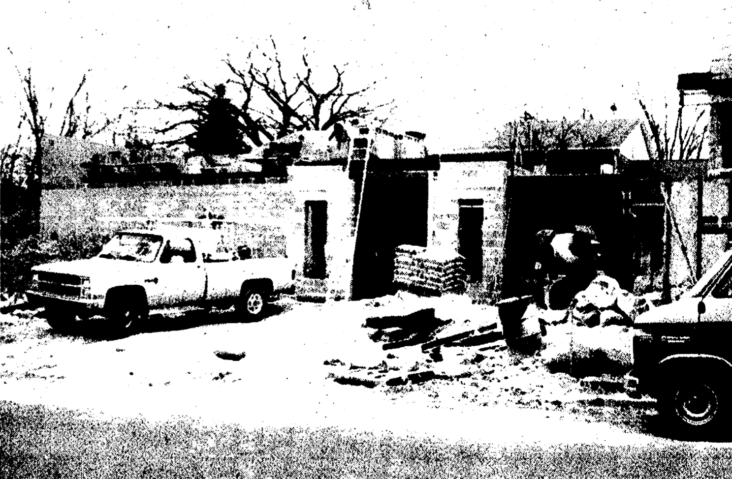
CONSTRUCTION is well underway on phase one of attached to the main church building, have offices, handicap access bathrooms, and other facilities. Methodist church on Park St. When completed it will be
